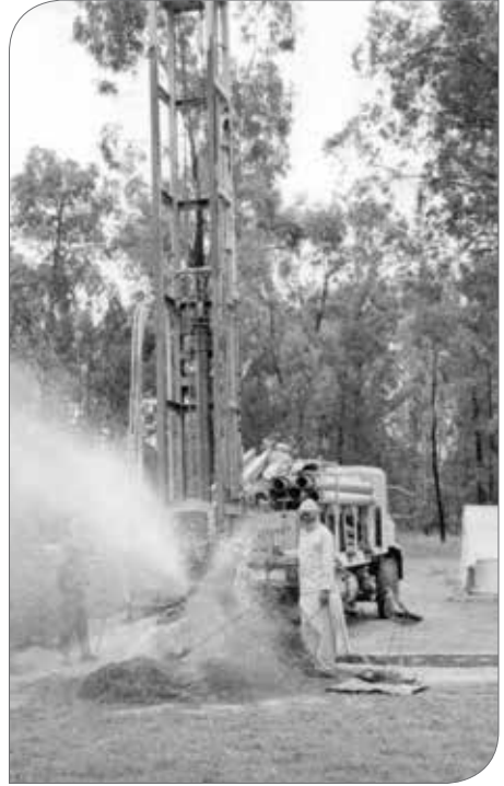
Drilling a borehole.
