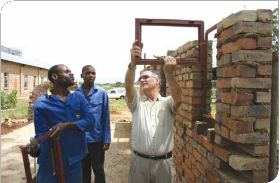
Mahube Valley: Fr Chico de Medeiros supervising the building of the toilets near the hall that functions as church (the parish house and catechism rooms were built later).
