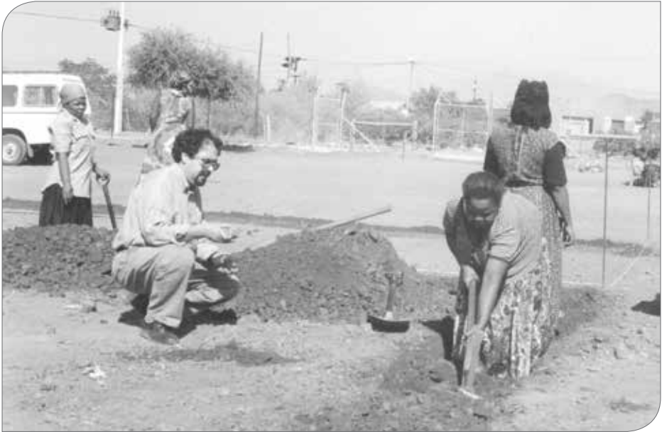
Bro. Artur Pinto supervising the work of opening the foundations for the construction of a church.
