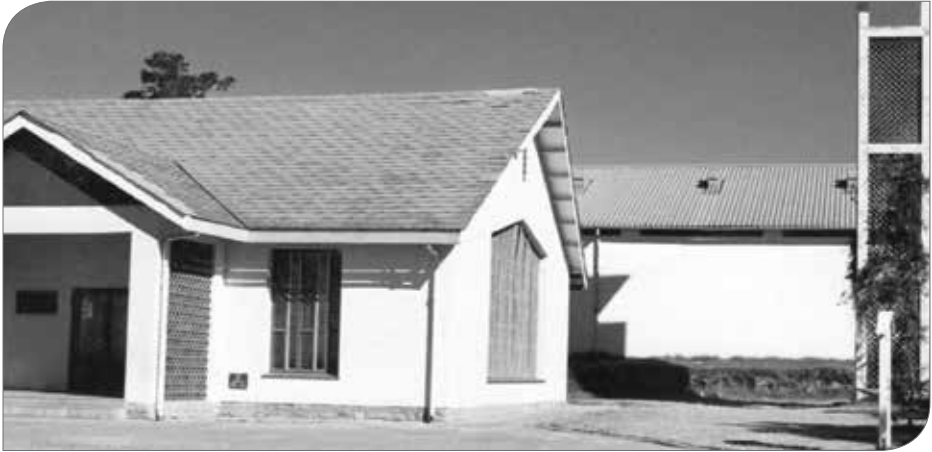
Parish buildings, in Mount Frère.
